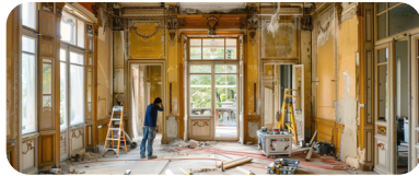
▷ Villa renovation and refurbishment
