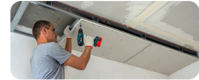
▷ Gypsum and decorative false ceiling works
