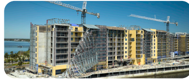
▷ High end residential building construction
